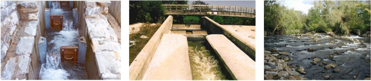
FIGURA 14: PASSAGGIO A BACINI SUCCESSIVI, PASSAGGIO DI TIPO "DENIL, PASSAGGIO A RAPIDA ARTIFICIALE
